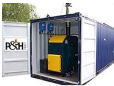
A single container installation – the fuel store is in the back of the container....
