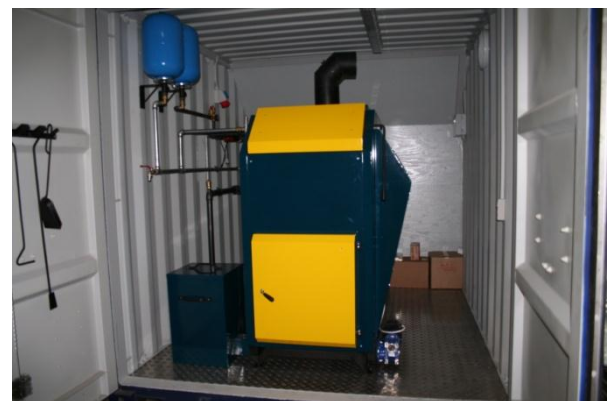
A dual container installation for a larger boiler – the lower container houses the boiler, the upper container is the fuel store.
