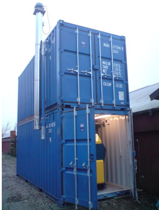
A dual container installation for a larger boiler – the lower container houses the boiler, the upper container is the fuel store.
